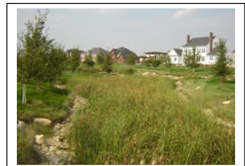
Figure 25: Example of a Drainage way
