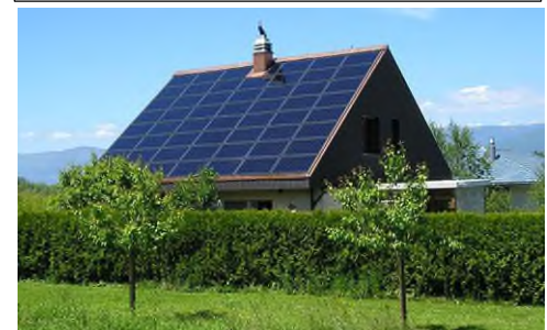
Figure 70: Example of a Solar Conversion System, Structure-mounted
